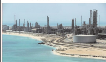
Construction site for an oil facility in Saudi Arabia.
