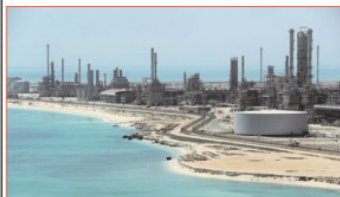
Construction site for the Saudi oil facility.
