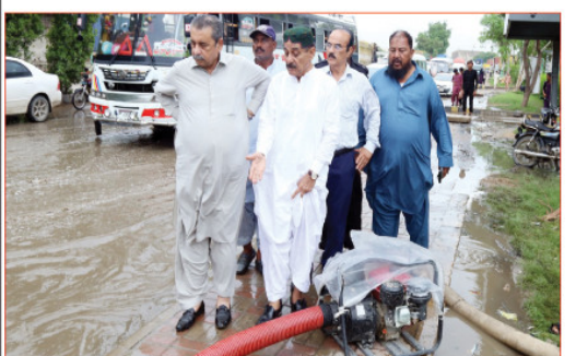
KARACHI: Advisor to the Sindh CM Syed Najmi Alam and Chairman of Malir Town Jan Muhammad Baloch are inspecting the rainwater drainage work on the National Highway near Popular Factory. —Photo by Asif Qureshi
